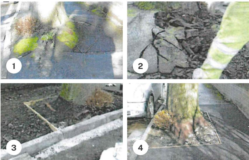
1. Before work showing humped tarmac and displaced kerb
